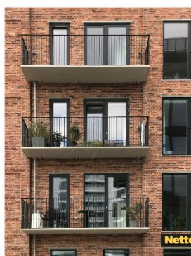
Spinkel altanbund i fiberbeton, Islands Brygge
