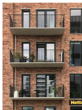
Spinkel altanbund i fiberbeton, Islands Brygge
