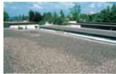
Soil and plants on a roof need not weigh more than a typical gravel roof – about 80kg per square metre.
