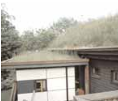
An extensive turf roof provides insulation for this London family house.
