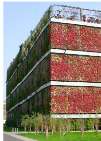
Grønne P-huse, High Tech Park, Eindhoven, Holland
